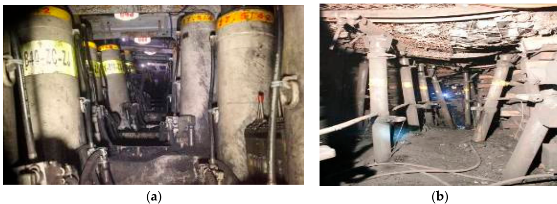
Figure 3. Strong strata behavior: (a) Crushed face supports; (b) Broken roadway pillars.
