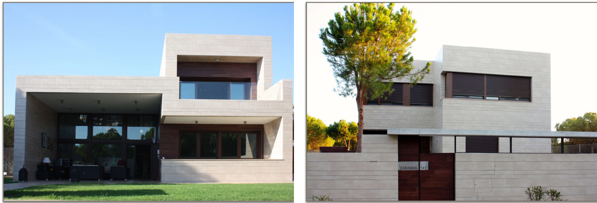
Figure 20. In the photo left and right , respectively: elevations south and north of Casa Zaranda. Final state.
