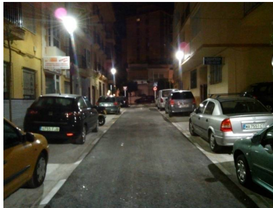
Figure 6. Spatial configuration of the luminaries related to the reference roadway of the field test in our study.
