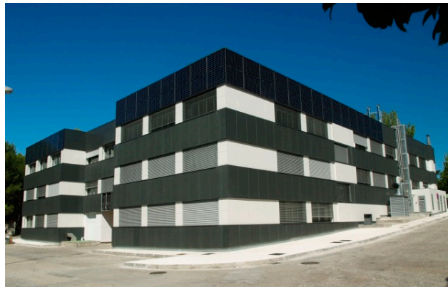
Figure 2. Southwest view of the building after the retrofit.
