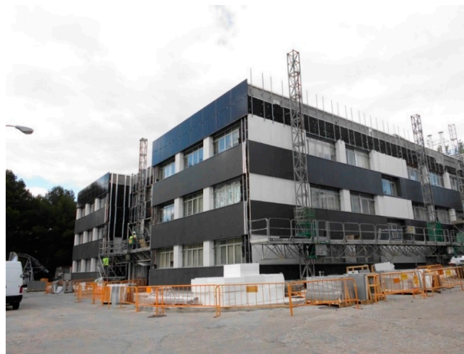
Figure 3. Southwest view of the rehabilitation works.
