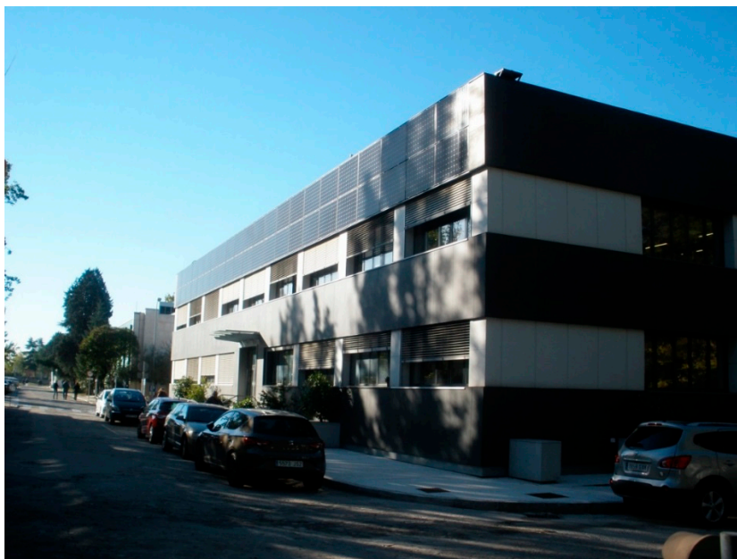
Figure 10. Partial shading by the trees of the east façade.
