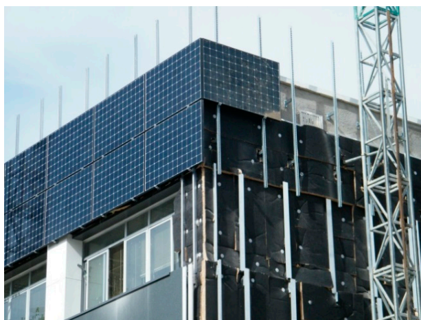
Figure 5. Constructive details of the PV modules fixation.
