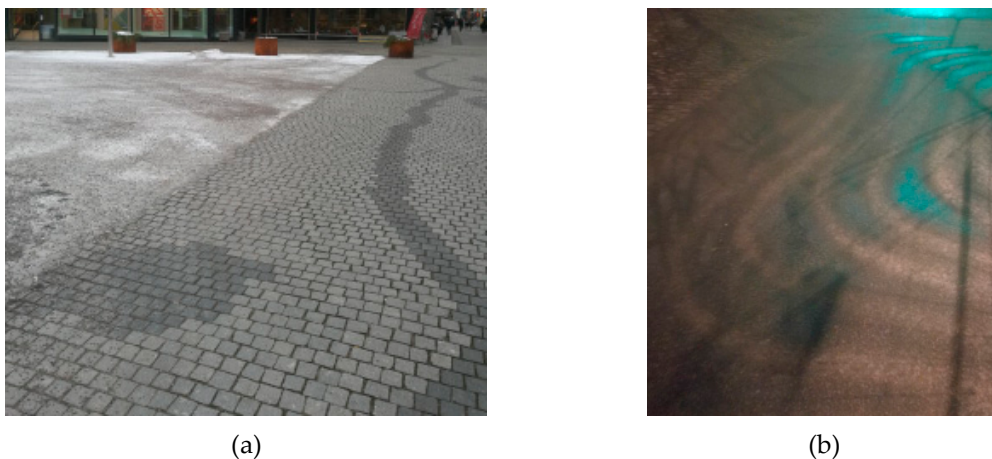
Figure 1. Pictures from the center of Linköping, Sweden. (a) A square at an outdoor temperature of -4 °C with an active hydronic pavement system (HPS) in the outer perimeter, plus conventional snow clearance and use of sand in the middle. (b) A walkway shortly after precipitation at 0 °C. The positioning of the HPSs embedded pipes can be discerned when the surface starts to dry up.
