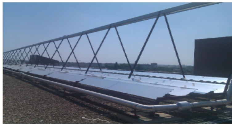
Figure 2. Fresnel collector field.
