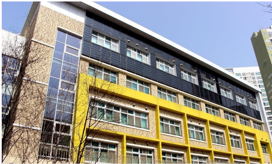
Figure 2. Demonstration building with air-type BIPVT collectors.
