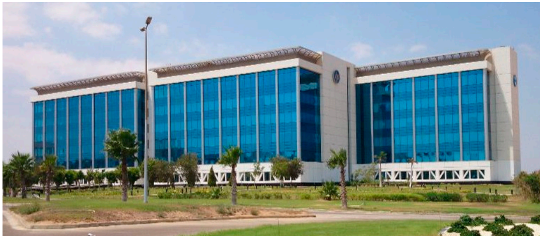
Figure 6. Building main elevation [16].
