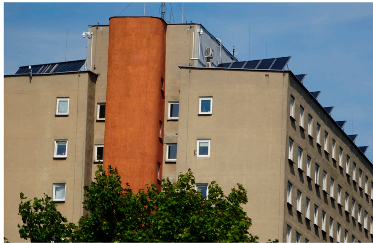
Figure 1. Solar domestic hot water (SDHW) system located on the roof of the 11-storey Bialystok University of Technology (BUT) hotel.
