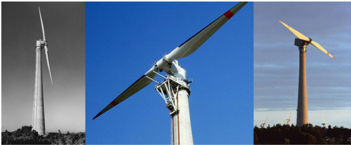
Figure 2. The Näsudden turbines. Left and center: The 2-MW Näsudden I (WTS-75) at Näsudden, Gotland. Photo used with permission from Vattenfall (left) and Jos Beurskens (center, all rights reserved). Note the lift platform that was used for erecting the nacelle, and thereafter the blades, during assembly. Right: The 3-MW Näsudden II at Näsudden, Gotland. Photo by and used with permission from Gunnar Britse.
