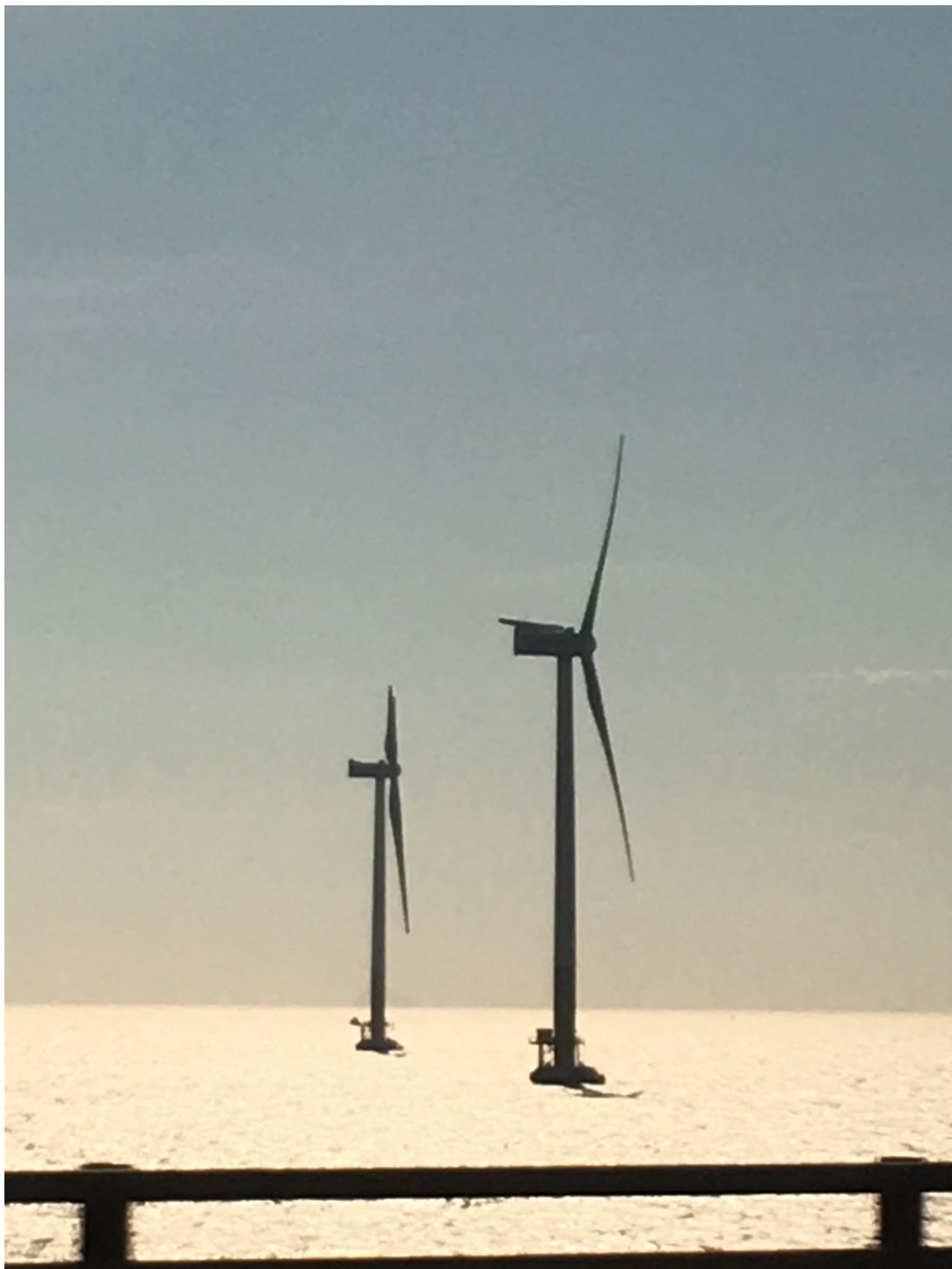
Figure 1. China's first off-shore wind farm in Yangshan Port.
