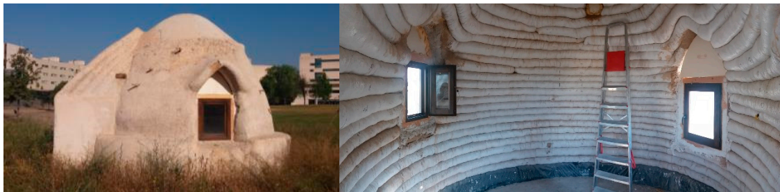
Figure 1. Earthbag building, University of Lleida Campus, Spain.
