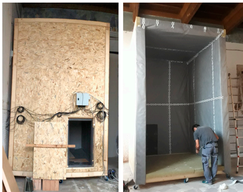
Figure 5. Box finishing: Thermal insulation and vapor barrier application.
