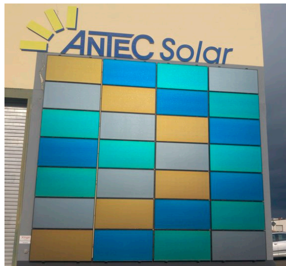
Figure 4. Multi-color solar wall Antec Solar headquarters in Arnstad Germany (source: [37]).
