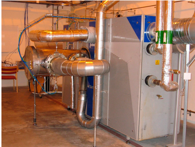
Figure 2. The MGT test rig.
