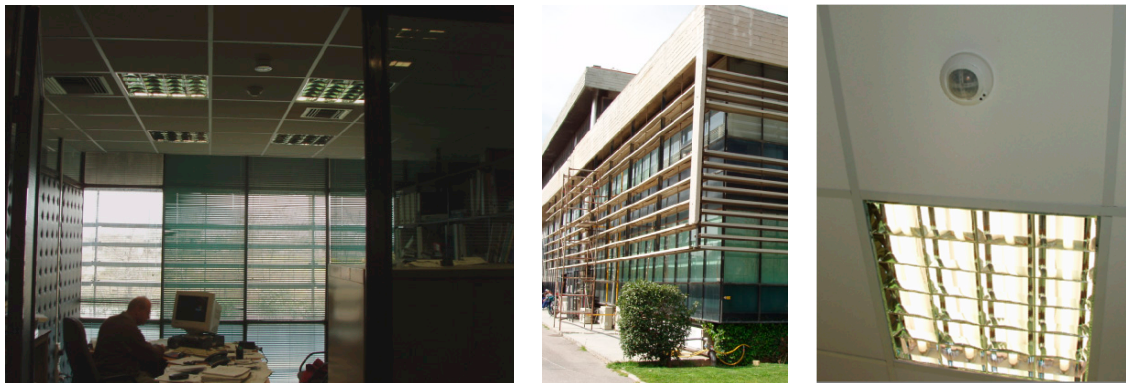
Figure 2. Interior space (left), exterior façade (middle) and position of the photosensor (right) for Building A.
