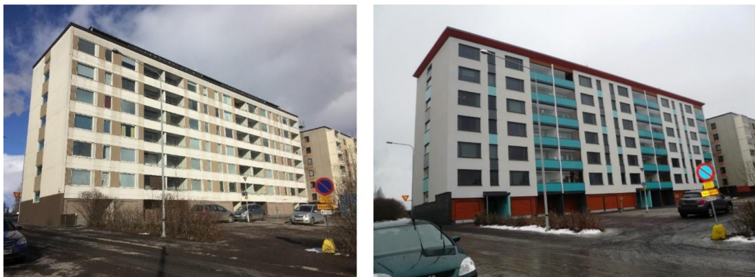
Figure 4. The studied building before and after retrofitting.
