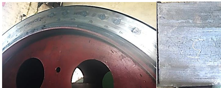
Figure 11. Surface damages of brake disc and brake shoe after emergency braking of coal mine hoist with high speed and heavy load.
