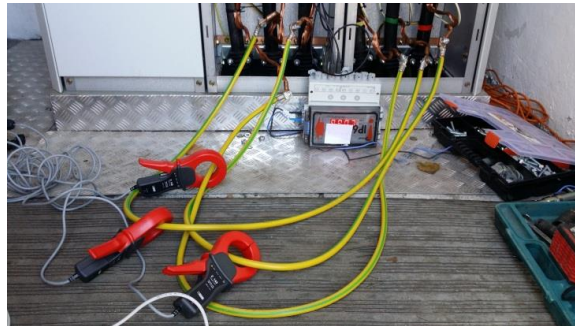
Figure 10. Sheaths unearthed and uncrossed in Substation 2.
