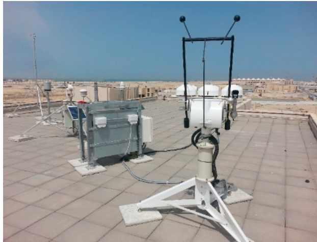
Figure 2. Solar monitoring station on the roof of the College of Architecture and Planning, Imam Abdulrahman Bin Faisal University, Dammam, Saudi Arabia.
