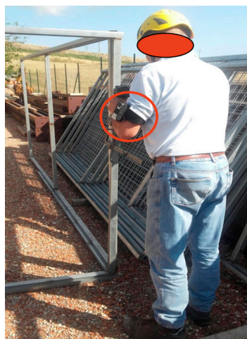
Figure 2. A construction worker in Tuscany wearing the GENESIS-UV dosimeter on the upper left arm.
