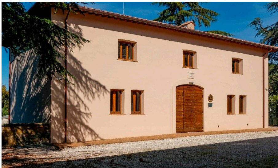
Figure 1. The case study building from the front side.
