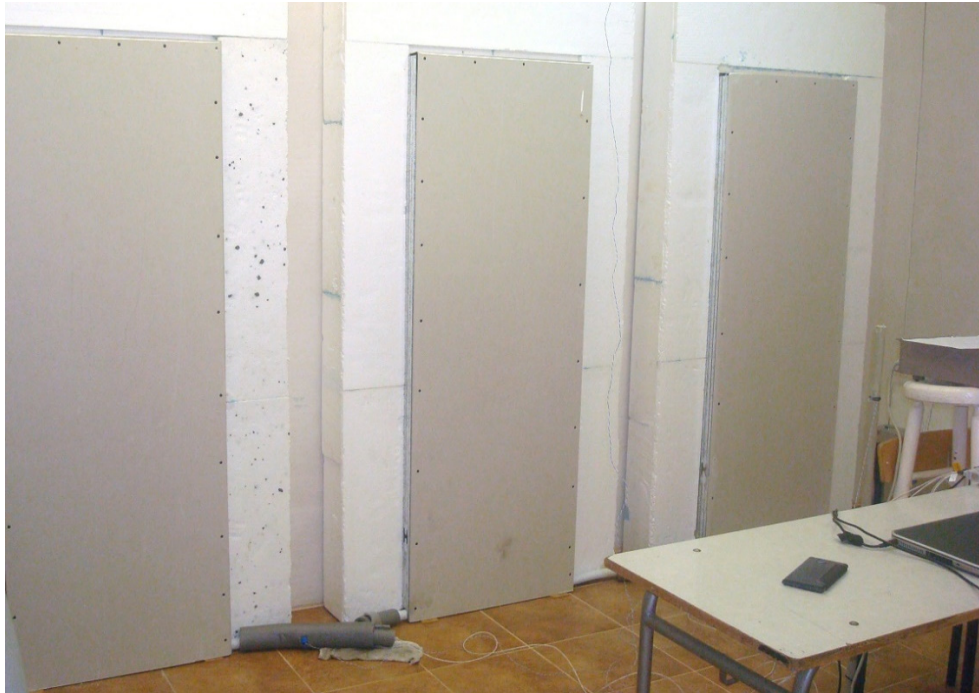
Figure 2. View of the investigated panels in the test chamber.
