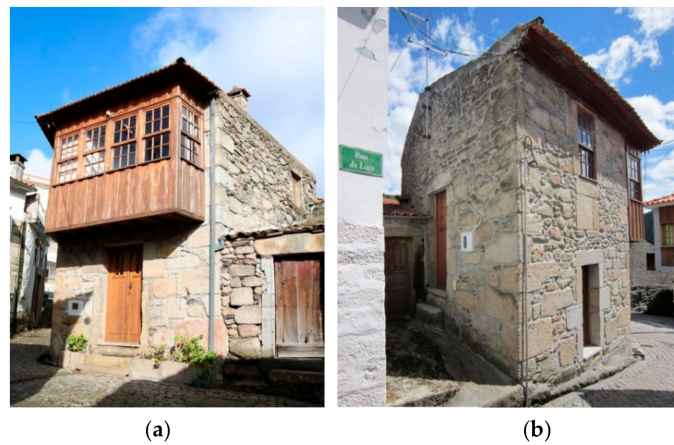
Figure 7. External views. (a) southwest and southeast façades; (b) northeast and west façades.
