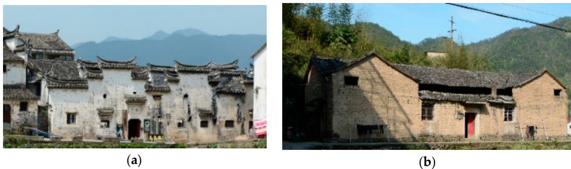
Figure 8. Exterior facades in (a) Heyang and (b) Danzhi.
