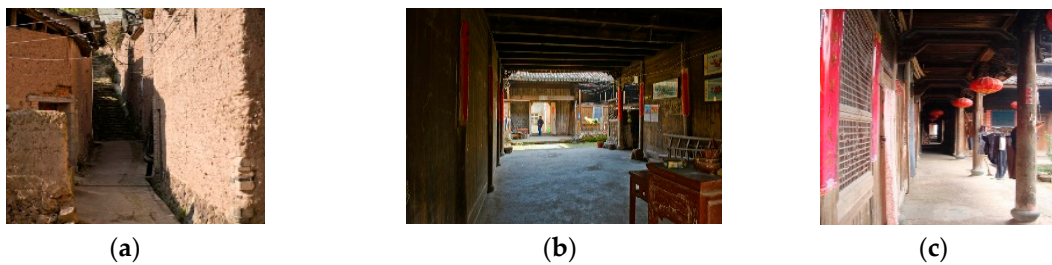
Figure 6. Typical (a) cooling avenue, (b) living room, and (c) corridor views of subject buildings.
