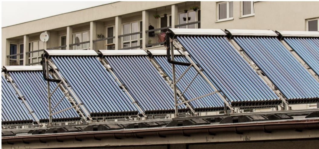
Figure 3. The ETC installation in Krosno.
