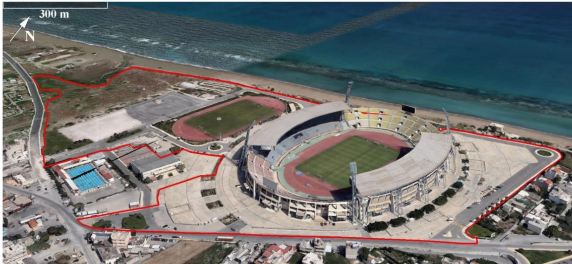
Figure 1. 3D representation of the Pancretan Stadium and the auxiliary outdoor space from southeast.
