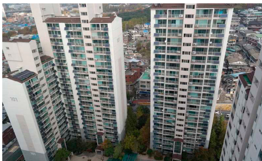
Figure 2. Installed mini-PV in Hongreung Dongbu Apartment buildings.
