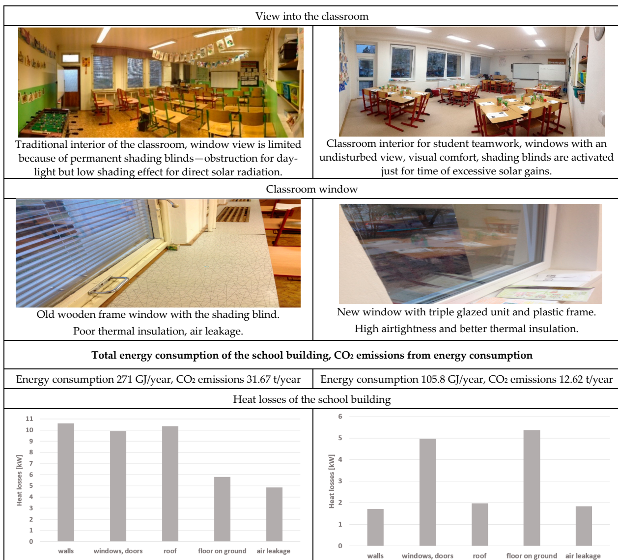
Figure 3. Photographs of the east wing of the school building campus with the classroom in its former and renovated states.
