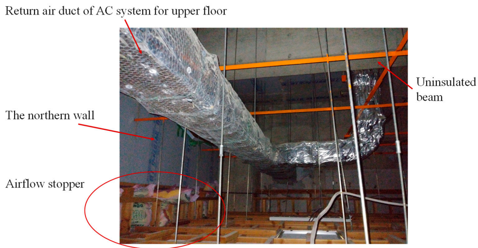
Figure 2. The duct passing through the attic space.
