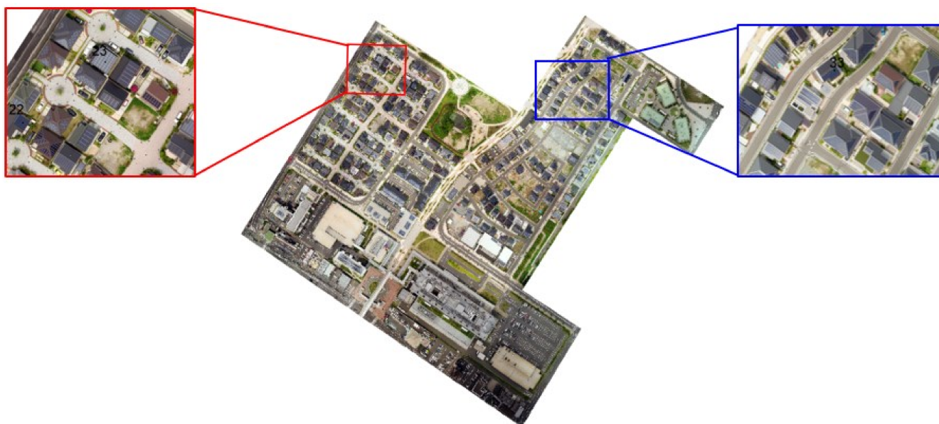
Figure 18. The high penetration of solar panels in the Jono residential area.
