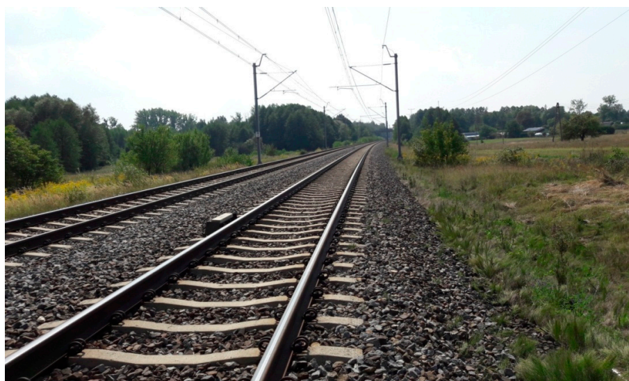
Figure 4. Railway track at km 18 + 600—experimental research area (curve).
