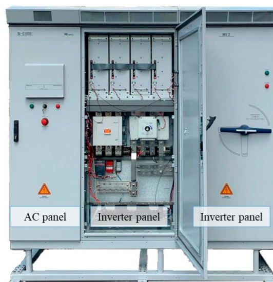
Figure 10. Image of the 1 MW PV inverter system.
