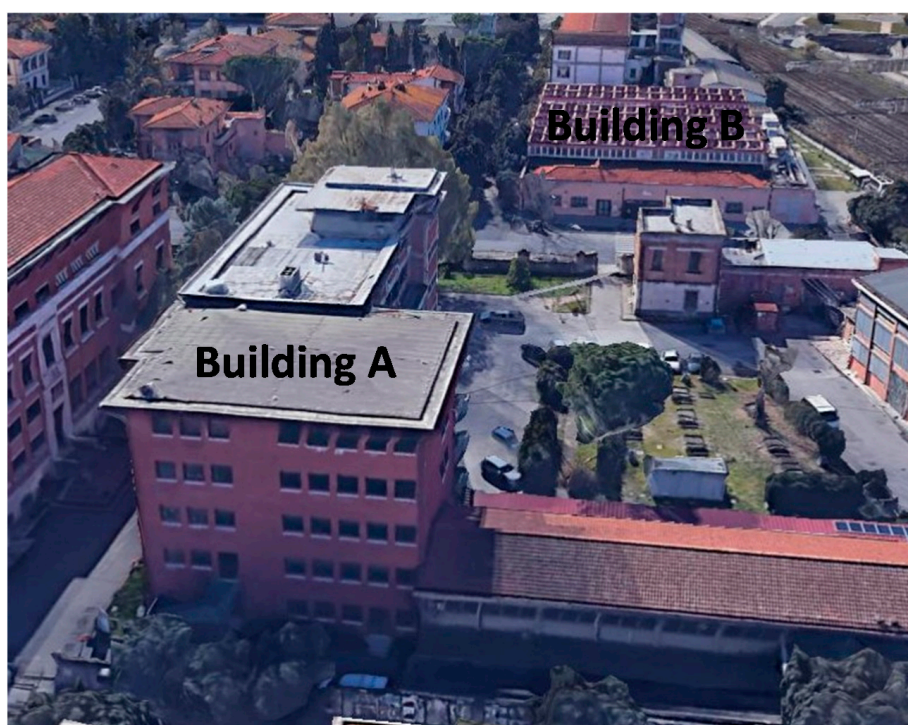
Figure 4. An aerial view of the two buildings, object of the analysis.
