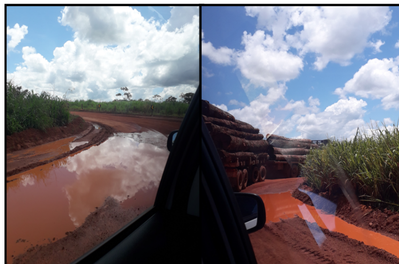
Figure 1. Poor road conditions in the Aripuanã region.
