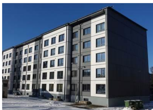
Figure 1. Overview of the nZEB case building after the renovation.
