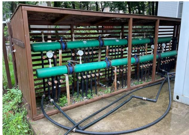
Figure 2. Water collector and separator device.
