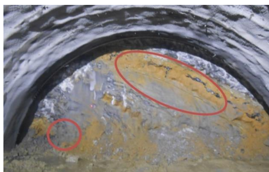
Figure 2. Water filtration at the front of the face.
