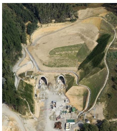
Figure 1. Tunnels under construction.
