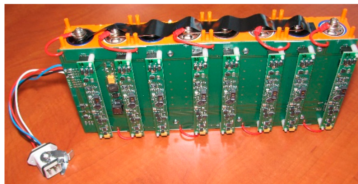
Figure 6. View of the active system (cell to battery) BMS installed on the cells package.
