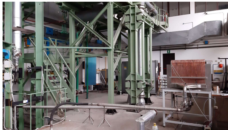
Figure 6. DEMO divertor OVT prototype installed into the CEF1 building.
