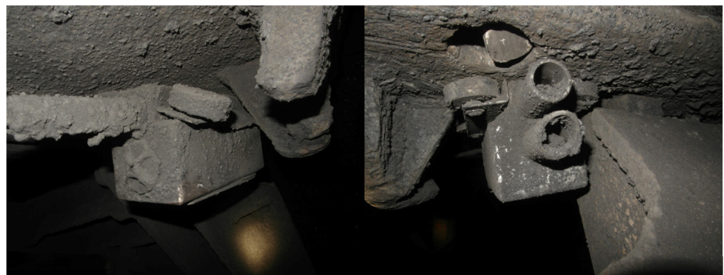
Figure 7. SSMS-S sensor in operation: harsh conditions.
