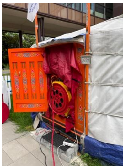
Figure 11. Blower-door fan installed in the external door of yurt.
