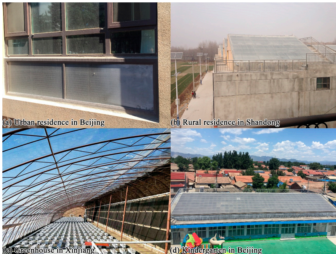
Figure 3. Construction projects using VTBC collectors.
