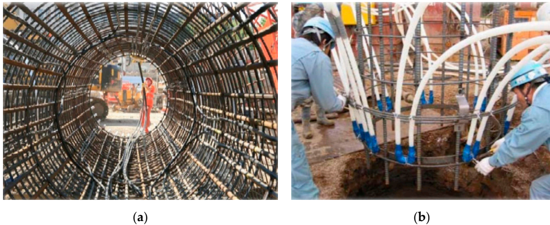
Figure 3. (a) The reinforcement of the energy pile, (b) the insertion of the reinforcement in the form of a basket equipped with a U-tube system into the borehole [52].
