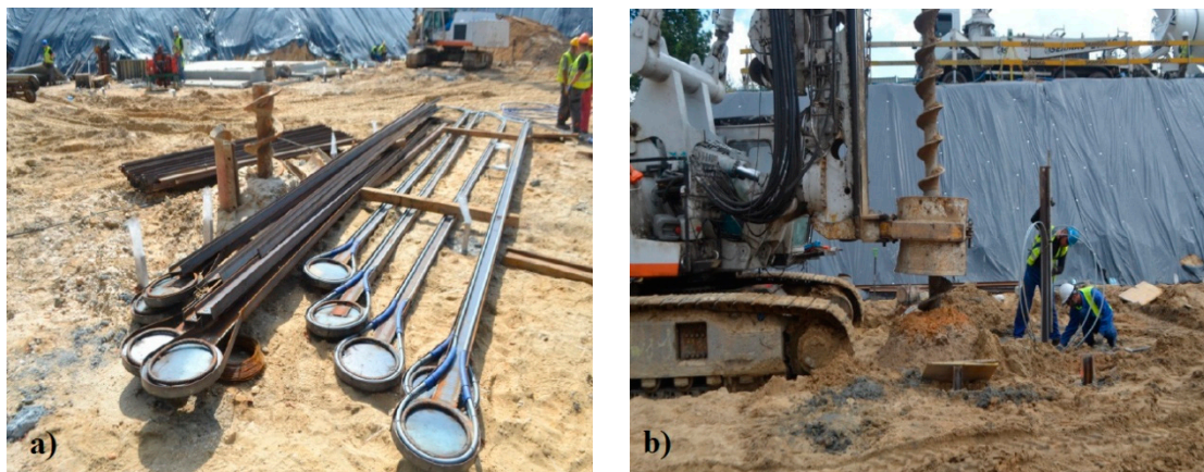
Figure 6. Execution of the energy piles in Krakow (the building of the National Archives), (a) reinforcement of the energy pile with an I-beam with a welded circular element, (b) execution of the energy pile.
