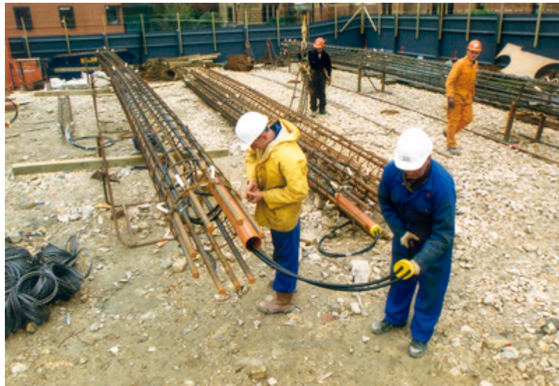
Figure 5. Laying the heat exchanger pipes in the load-bearing pile structure [55].
