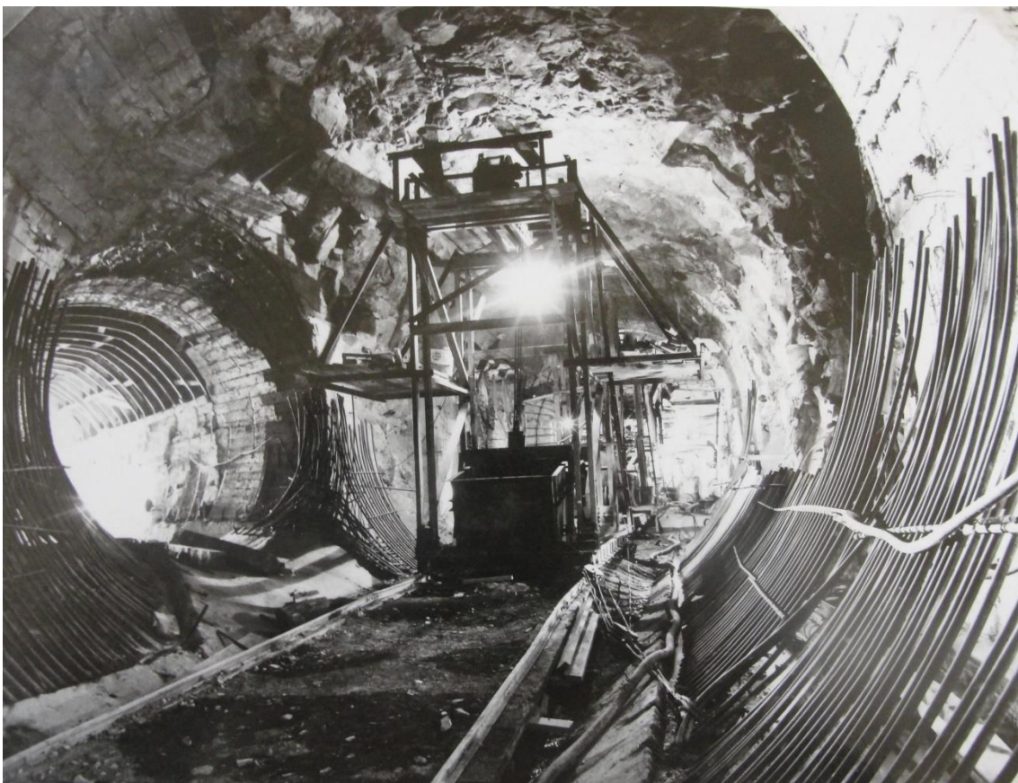
Figure 2. Construction of the power tunnels of Hirfanlı Dam—Turkey [3].
