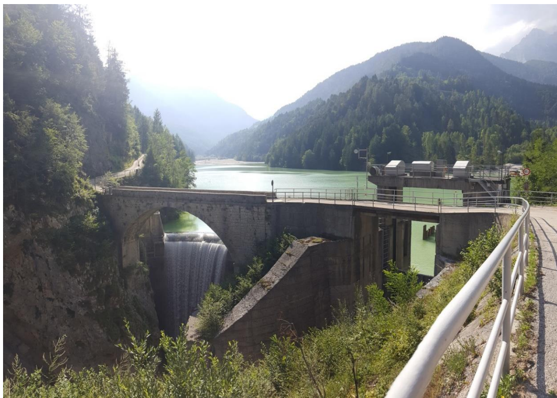
Figure 7. Valle di Cadore Dam—Italy (photo taken by the author on 11 August 2019).
