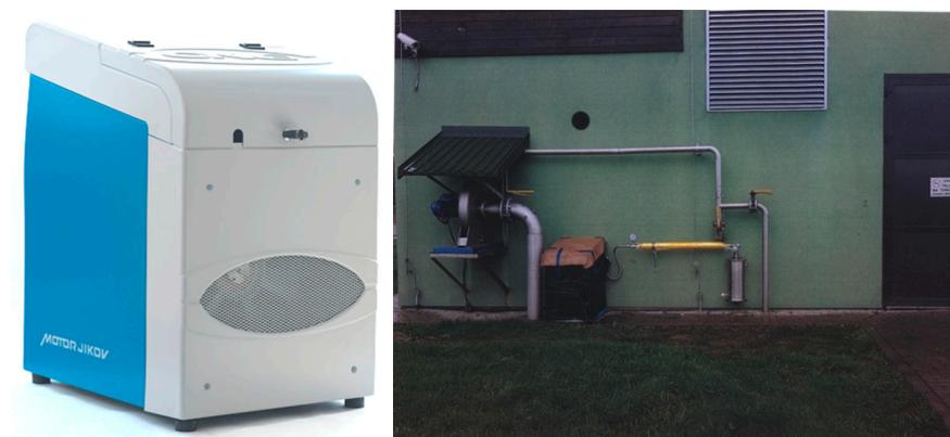
**Figure 8.** Gas compression station—view of the gas installation. Gas compressor with a maximum power input of 2.5 kW and a nominal capacity of 5 m<sup>3</sup>/h (at 15 °C, 200 bar, at 0.1 bar gas pressure at the inlet) (resources of the Institute of Technology and Life Sciences).
