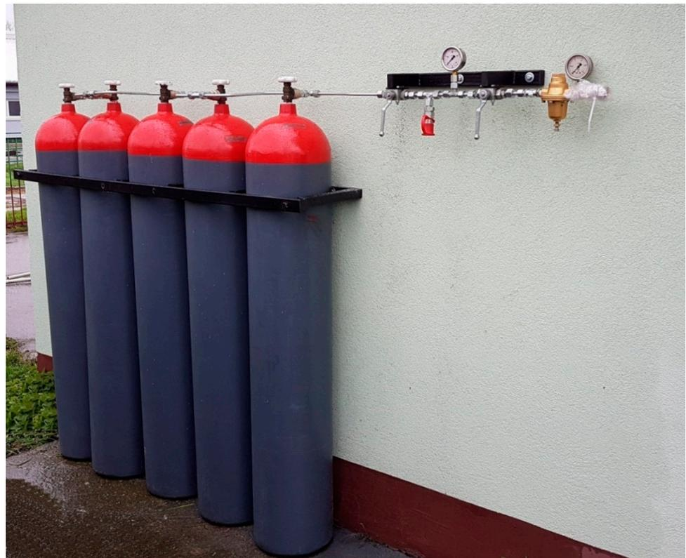
**Figure 9.** View of cylinders connected for the biogas system in the installation in a piggery in Jaworze (archives of the Institute of Technology and Life Sciences).
