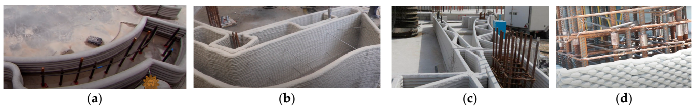
Figure 8. Reinforcement strategies for 3DPC used in on-site building constructions: (a) vertical rebars tied by a curved horizontal rebar in a curved wall element (ICON [59]), (b) vertical rebars with form ties in a wall element (CyBe [57]), (c) concentrated reinforcement in a wall element (Apis [58]), and (d) concentrated reinforcement connected by rebar couplers in a column element (WinSun [60]).
