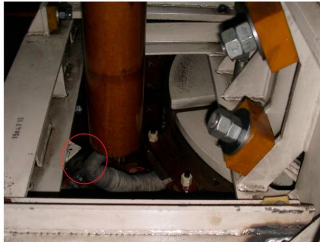
**Figure 10.** Identified ‘source’ increased discharge activity (Highlighted in a red circle).
