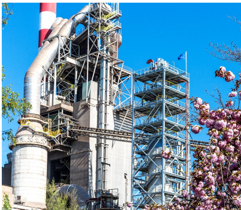
Figure 2. Picture of the LEILAC I reactor in Lixhe cement plant in Belgium Picture credits: HeidelbergCement/Paul Poels fotografien, Meerlo, NL.
