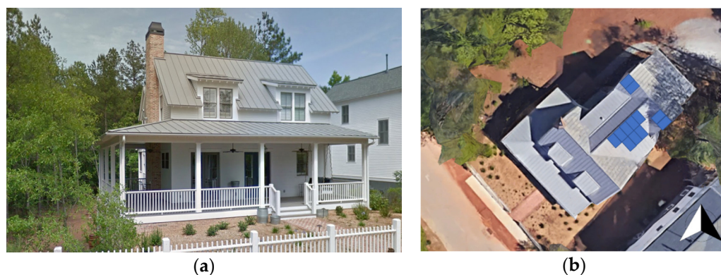
Figure 6. Building C in the Serenbe Community. (a) Front view (southwest); (b) roof view (PV covers 10% of the roof space). Source: modified from Google Maps 2021.
